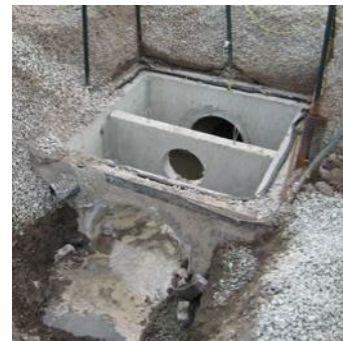
Figure 3-1 Outlet Control Structure, ARC, Wilmington,
