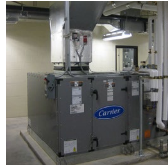
Figure 3-11 Air Handling Unit
